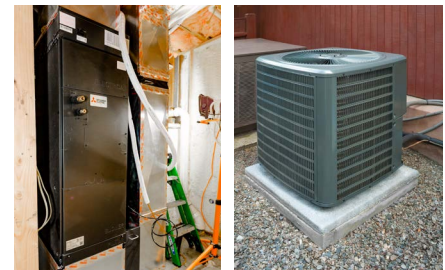
DUCTED ASHP, WITH INDOOR AND OUTDOOR COMPONENTS.
